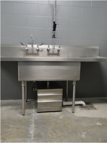
Root Washing Facility
